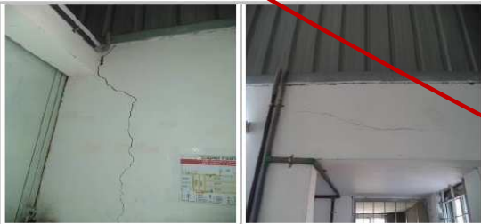
Cracks in walls
