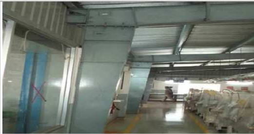
PEB shed without vertical bracing
